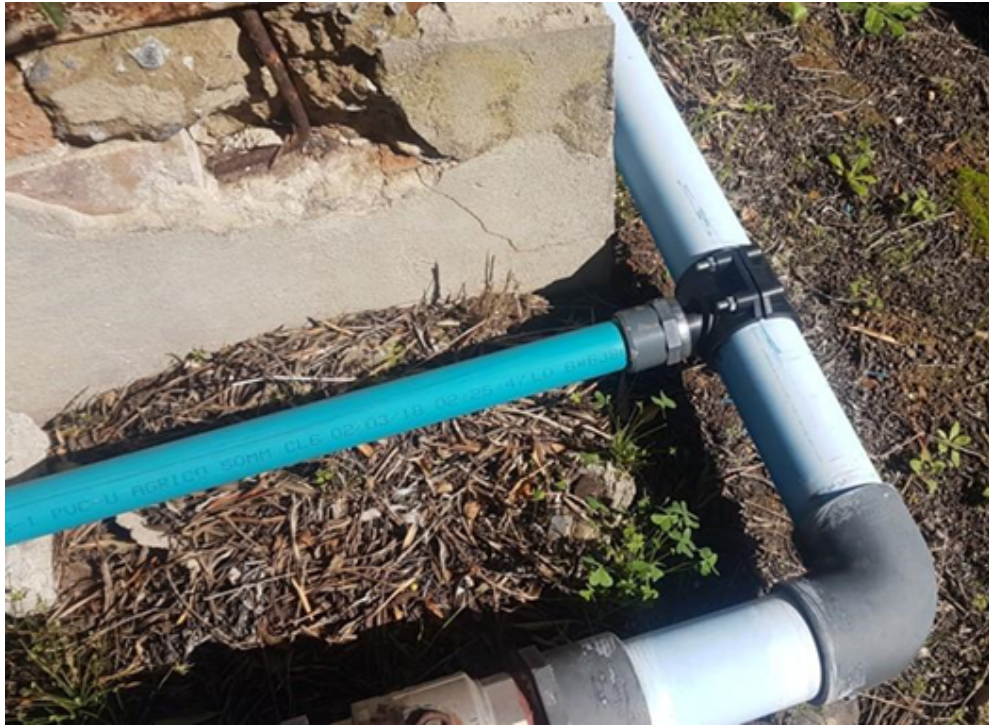
Figure 17. An image of the connection in the extraction pipe between the reservoir and the existing pump used to irrigate vineyards on the Welgevallen Experimental farm.
