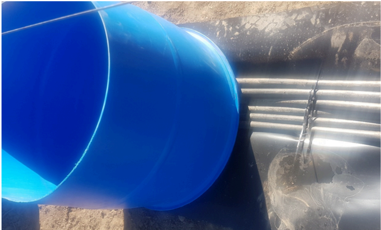
Figure 10. A 105 L PVC pot is placed on top of dpc and irrigation pipes.
